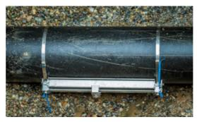
8 Position the ultrasonic sensors in the mounting rail and tighten. (The exact position in the rail depends on the pipe attributes.)
