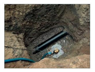
Cost-effective installation without chamber construction
